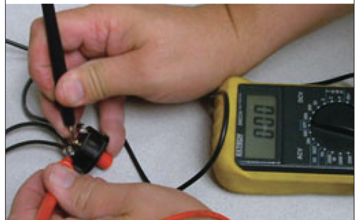
Figure 24. Testing Overload Protector
